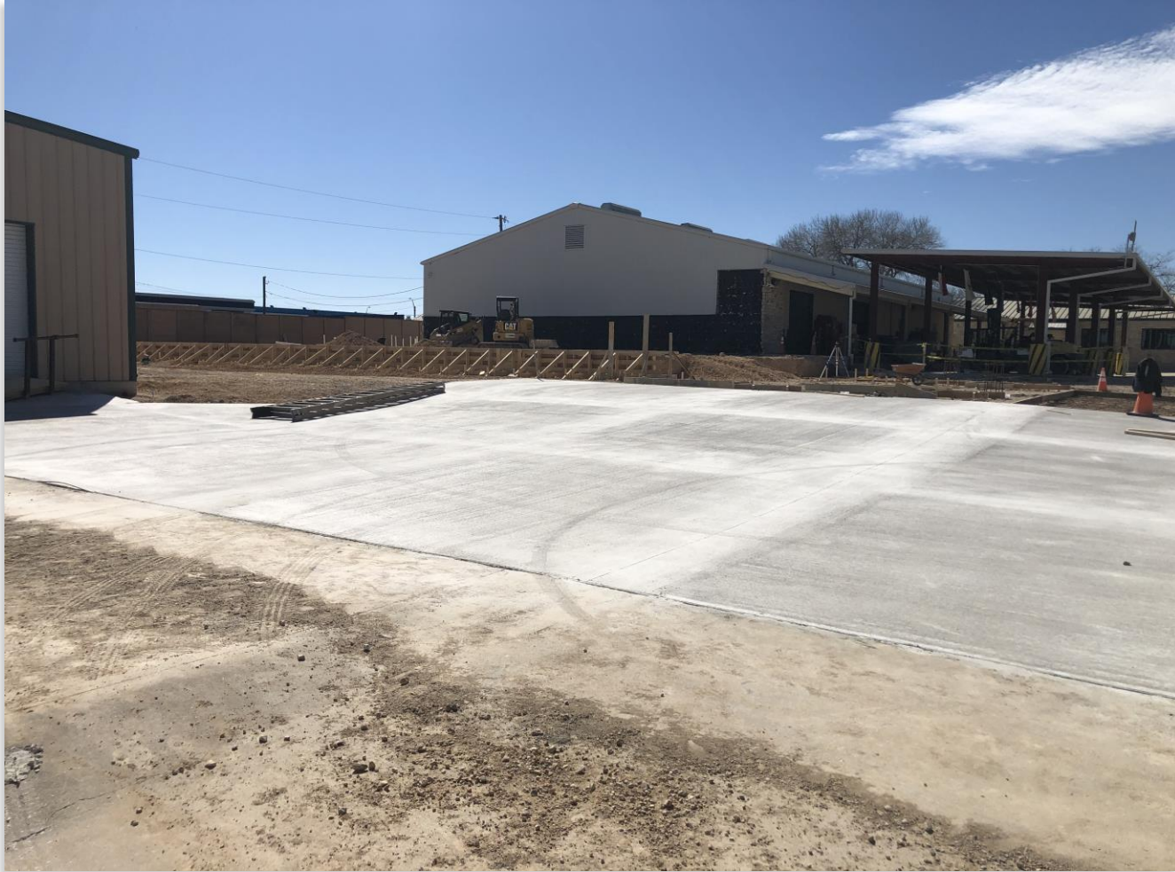
Warehouse Slab Preparation
