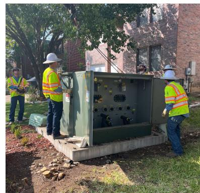
JSSO (Job Site Safety Observation) for an Oak Hill maintenance crew supervised by Benjie Juarez, was tasked with changing out an oil-filled switchgear.
